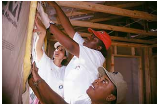
Volunteers put up insulation in a Habitat house in Plains, Georgia.
