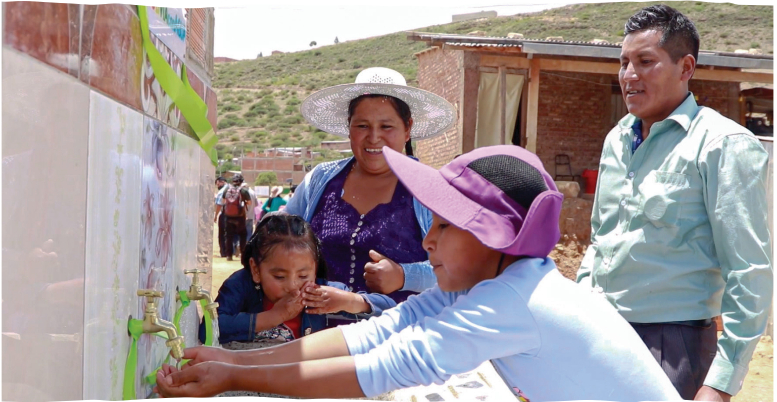
A Bolivian family uses a sink that was installed in their community. / Habitat for Humanity Bolivia.
