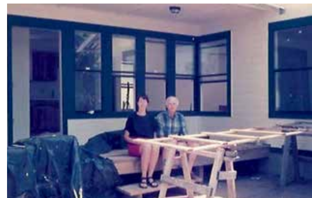
Maureen and her father, Henry Diercxsens, on site of the Habitat house that she designed and helped build 20 years ago. Maureen’s son, Taylor, is helping to build a Habitat home (above) in her honor.
