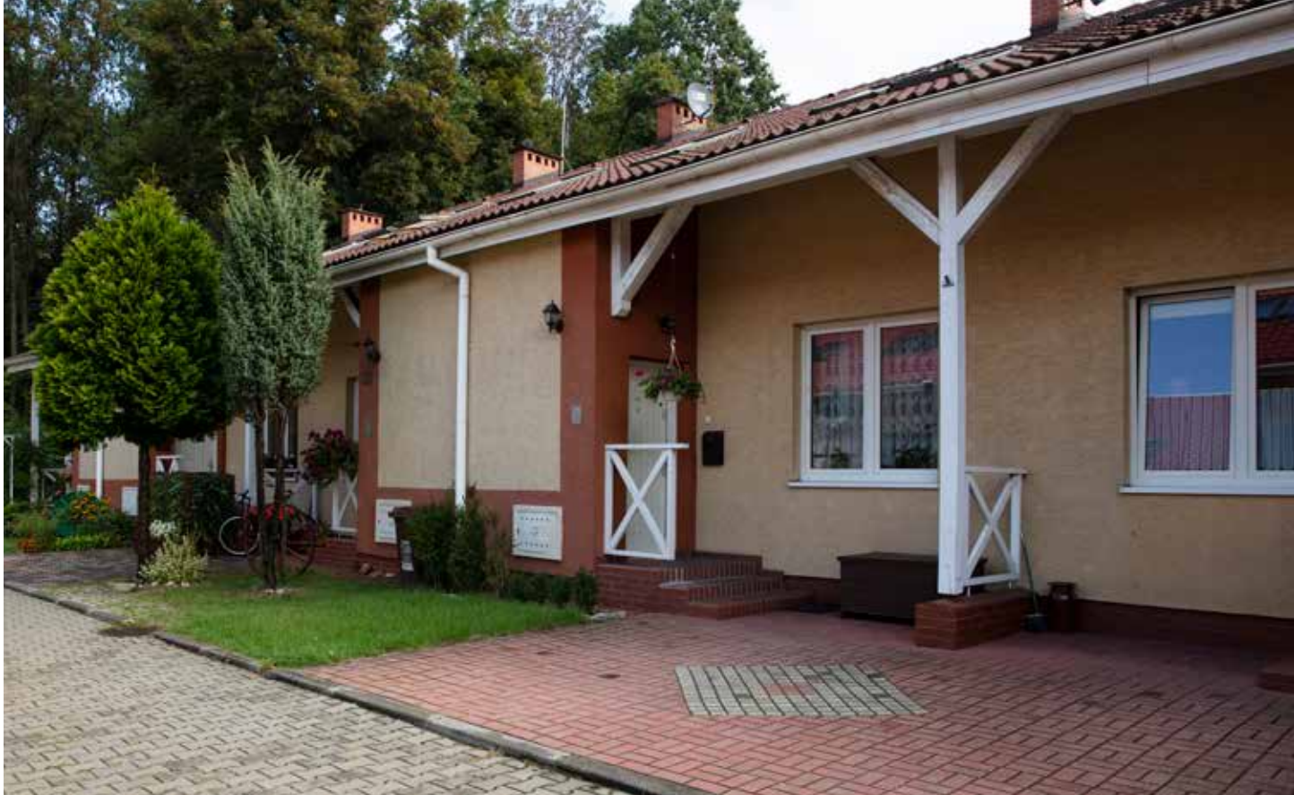
These rowhouses were among the first homes built by Habitat Poland.
