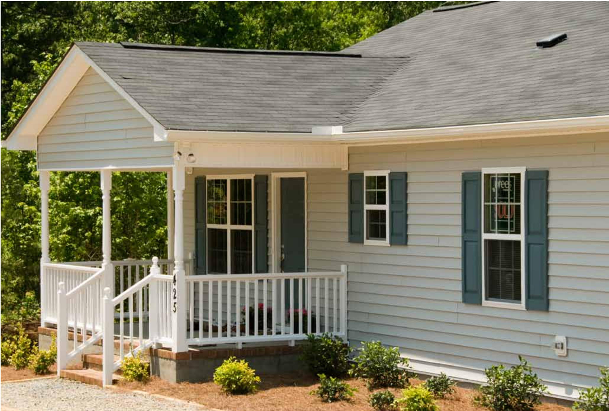
This Habitat house was built by local builders who volunteered for the Orange County, N.C., Habitat affiliate during a national "Home Builders Blitz."
