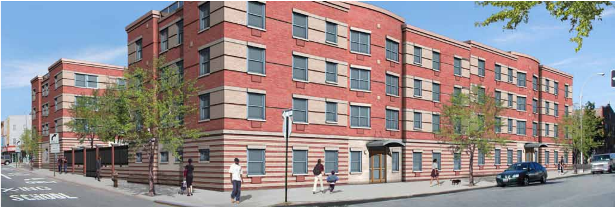
Multi-family complexes are often built in cities and suburbs; this project will be home to 41 families in Brooklyn, N.Y.'s Ocean Hill-Brownsville neighborhood. It's one of the largest, and greenest, complexes ever built by a U.S. Habitat affiliate.
