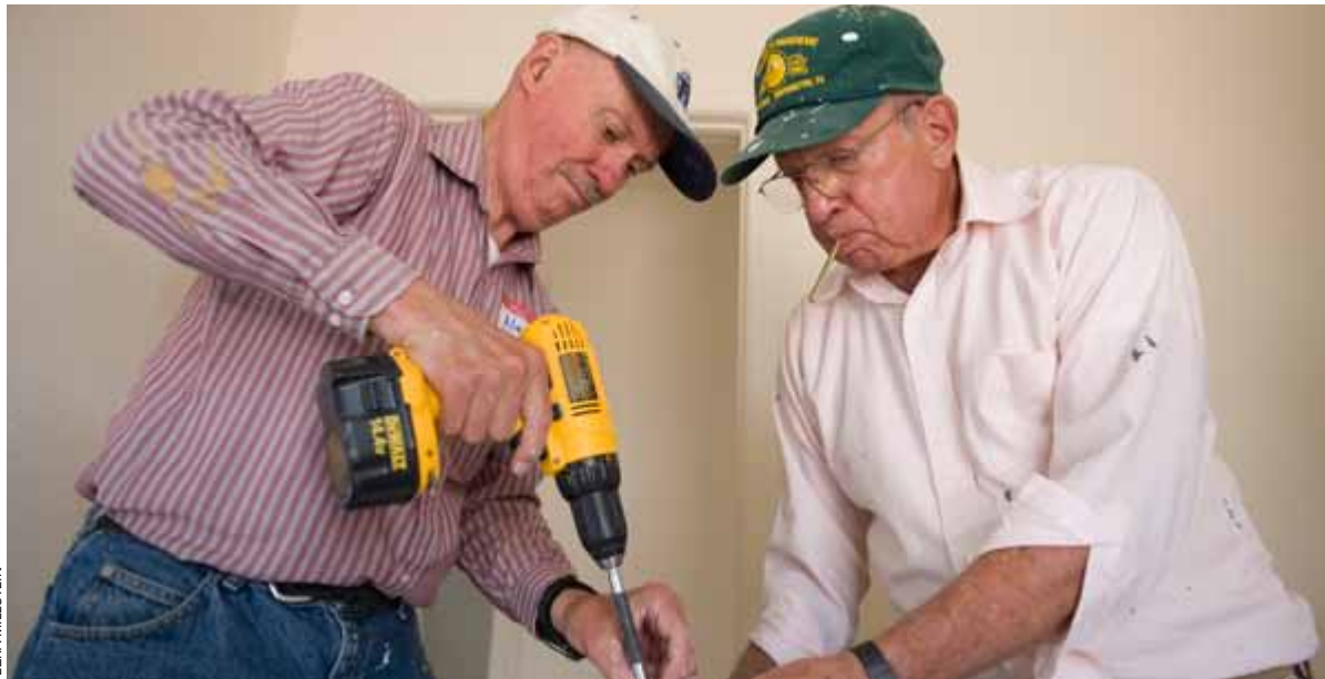
Volunteers Alex Zimmerman (left) and Hal Arner from Albuquerque, N.M., install a door in a new Habitat home.
