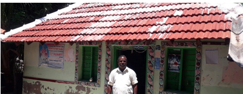
Amuthavalli's house after the new roof was installed.
