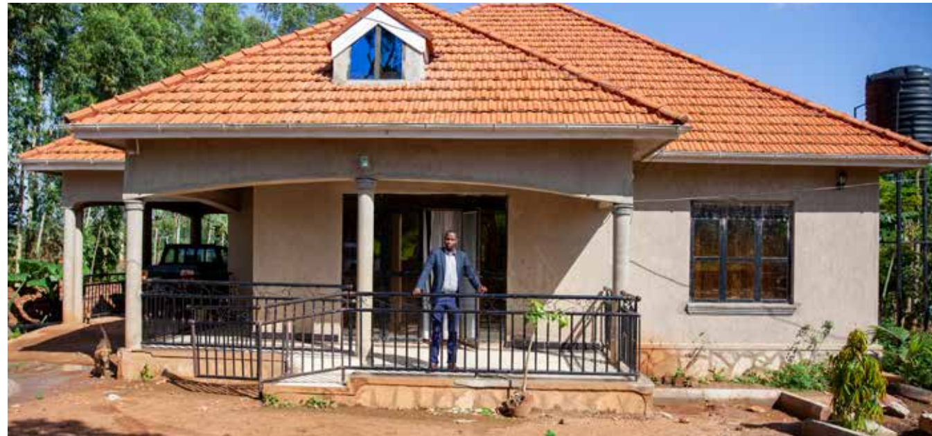
Dan saved money for many years to buy the land and lay the foundation for his home.
