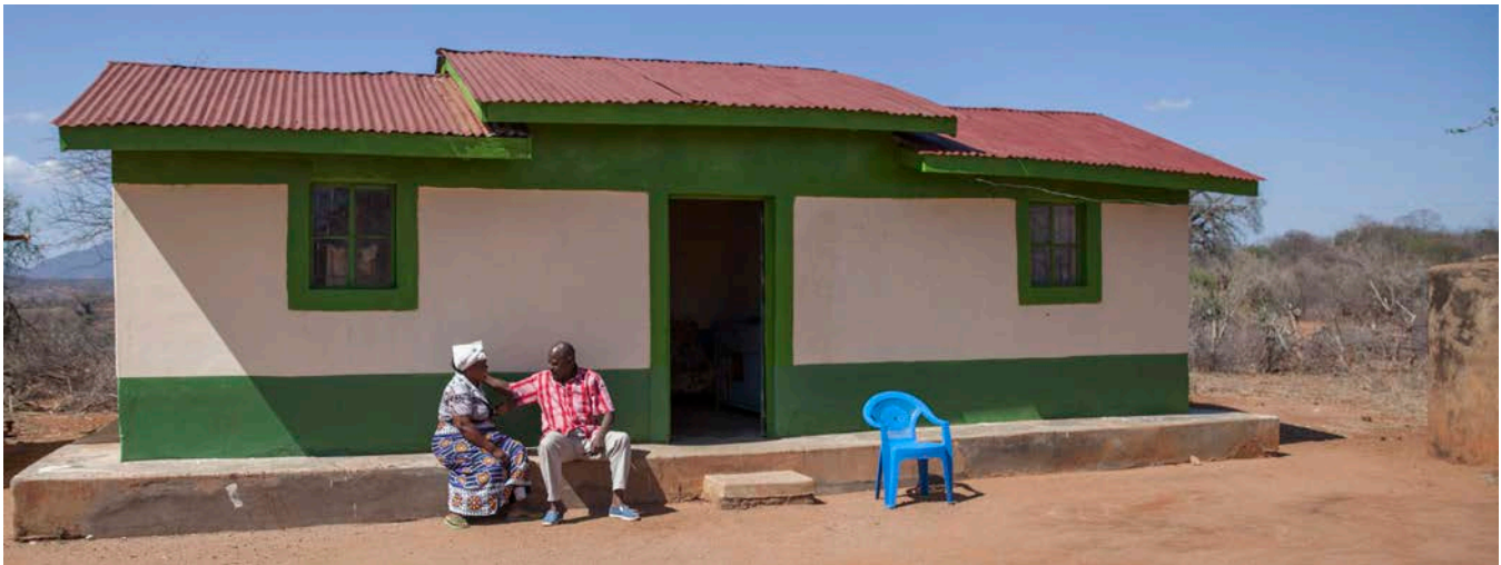
The Nyumba Smart Loan helped Annah and her husband complete their house, including installing a decorative steel door.
