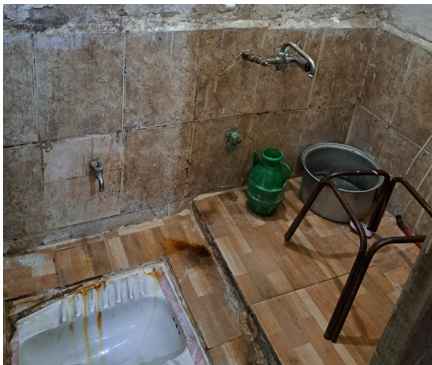
Before-and-after pictures of a sanitation facility in a Habitat-renovated home in south Amman, Jordan.
