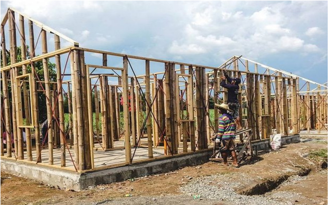
Base Bahay Foundation Inc.'s Cement Bamboo Frame Technology is a prefabricate bamboo building system designed to be earthquake resistant
