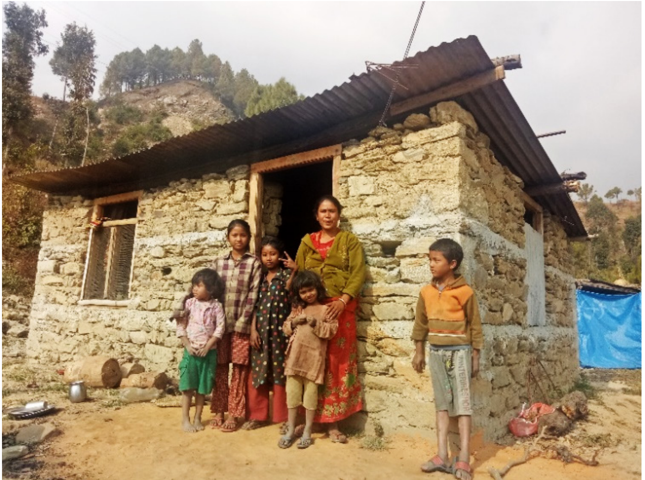
Family in front of reconstructed house. The new house is small and single story; the destroyed house was large and double-story, Rasuwa 2018. © Housing Recovery and Reconstruction Platform.
