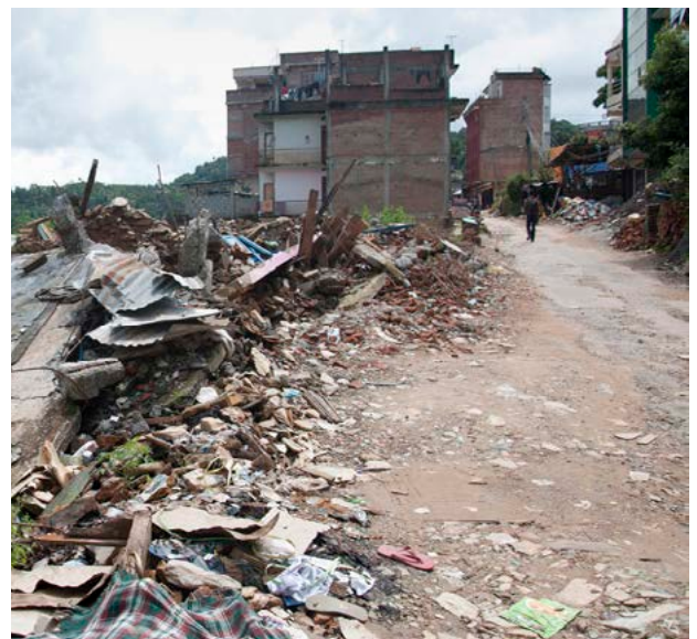
Destruction of secondary towns in rural districts.
