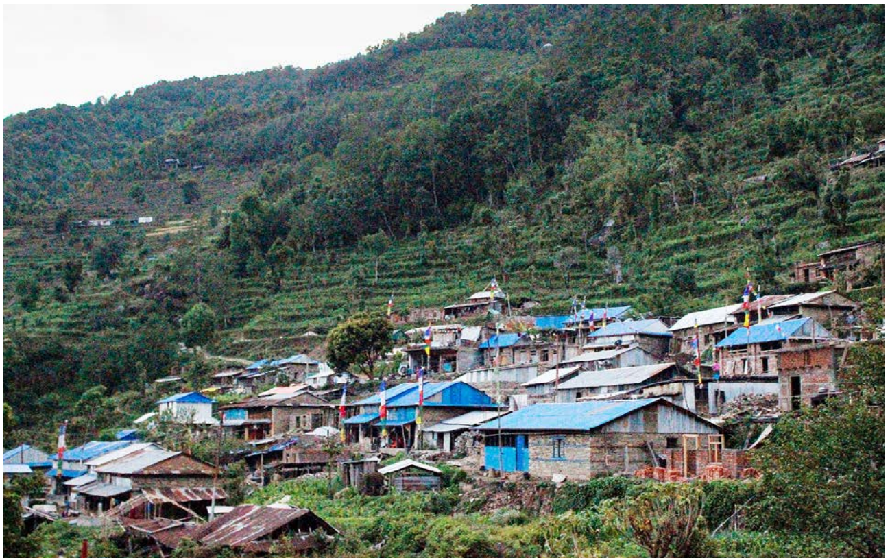
Housing reconstruction after the earthquake Salme, Ghalegaun. © Habitat for Humanity Nepal.
