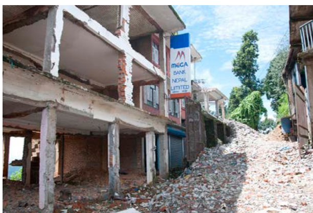
Streets in Chautara blocked with building rubble after the earthquake, 2015.
