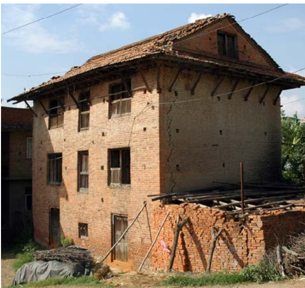
Typical brick multi-story house type, prevalent before the earthquake.
