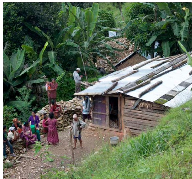
Shelter constructed by family using salvaged stone and new CGI roof sheets, 2015.
