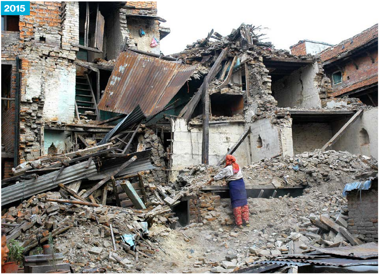
Local residents dismantling damaged buildings, 2015, Bhaktapur.
