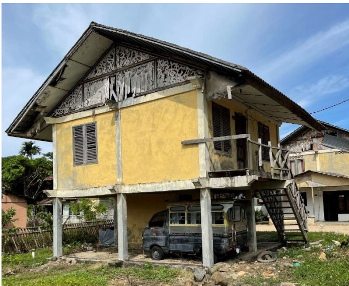
Figure 5. Elevated house with reinforced concrete posts, concrete walls, and timber flooring
