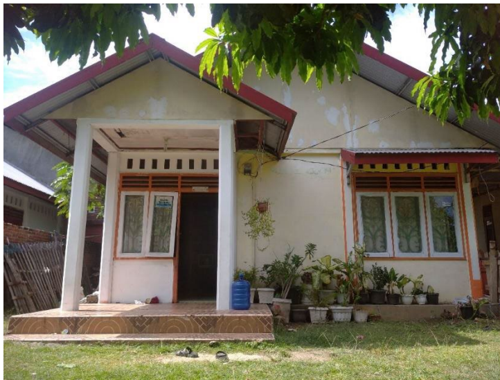
Figure 7. Single story with prefab concrete panel walls house
