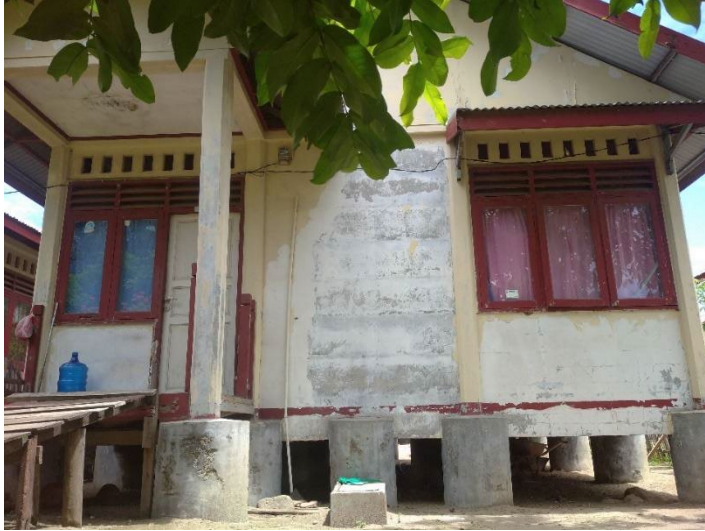
Figure 6. Elevated single story with prefab concrete panel walls house
