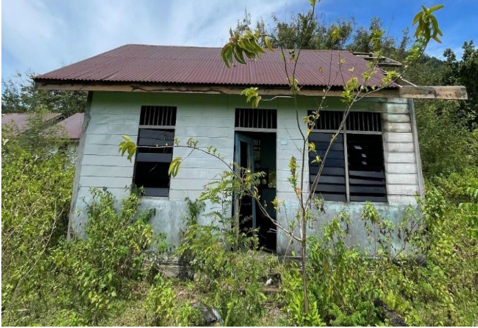
Figure 4. Single story with Kalsiboard walls house
