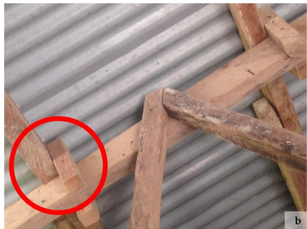
Figure 10: Examples of purlin-truss connections. a) A wind strap is used to connect the purlins to the truss. b) Wooden cleats are used to connect the purlins to the truss.
