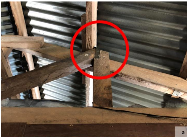
Figure 10: Examples of purlin-truss connections. a) A wind strap is used to connect the purlins to the truss. b) Wooden cleats are used to connect the purlins to the truss.
