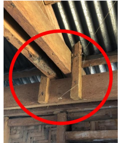
Figure 11: Truss-wall connection in Community C wooden shelter.
