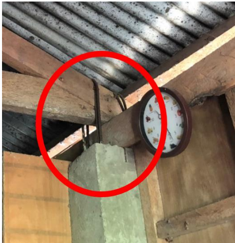
Figure 13: Example of wrapped rebar connection.
