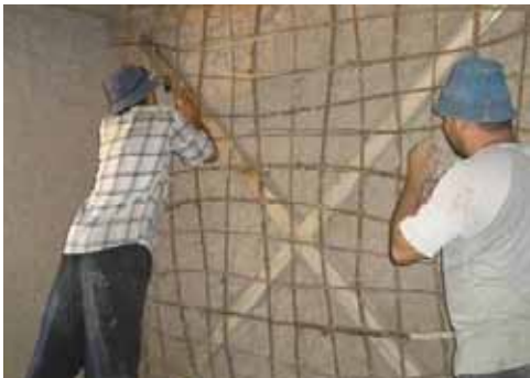
Masons in Tajikistan reinforce mud walls with mulberry tree branches.
