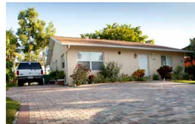
This Habitat home in Naples, Florida, was built with help from NSP2 funds.
