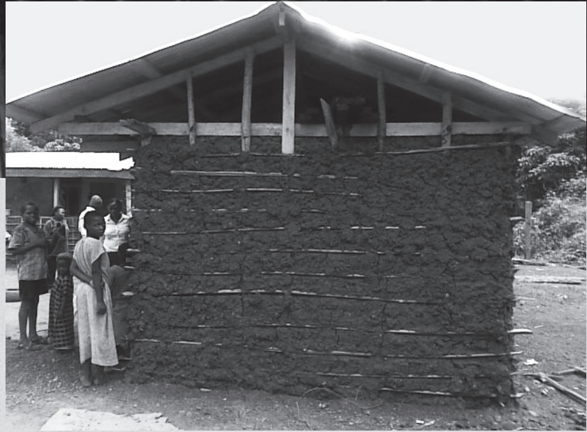
A microfinance loan study in Ghana involving improvements done without construction technical assistance revealed that this home received a new roof improperly placed on a structure of mud walls that cannot properly support the addition. The home could collapse, the study said, or the roof could be blown off during a heavy storm.
